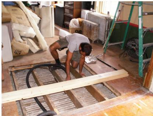
Left: preparing for the lift shaft.
