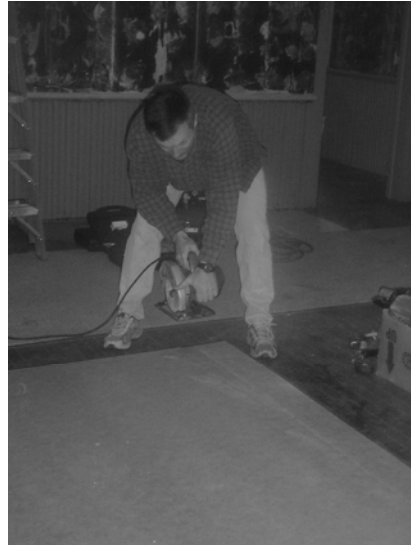
Steve Myers, historical society volunteer, cuts the first of 20 pieces of masonite hardboard that will become the new blackboards in both first floor rooms of the 1889 Cedarville school. The smooth side of each board will be finished with a special paint.
